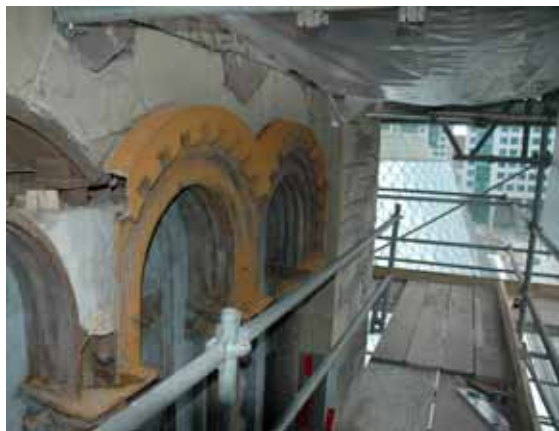
Left: Metal components on the West Tower, which look like stone from street level.
