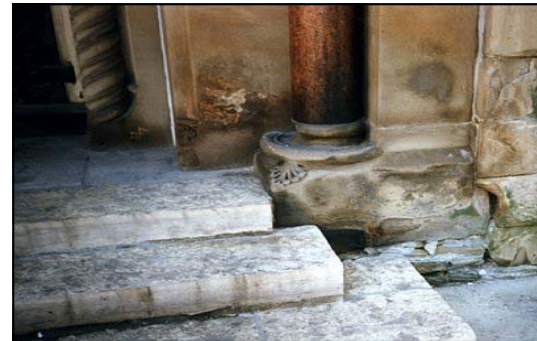
Left: Restoration work begins--as seen from Pat and Eric Reynolds' condo in Symphony Place. Right: Photo from the 2003 Capital Campaign showing the extent of the deterioration of the base of columns and building.
